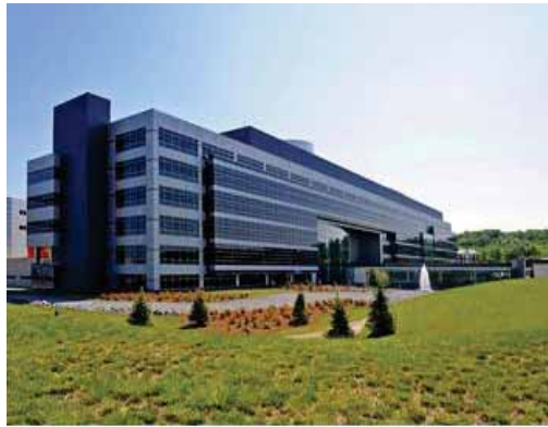
Fig. 4. The building of a new wing headquarters DIA, Anacostia-Bolling, SmithGroup JJR design, 2005. Source: Wikipedia Commons.
